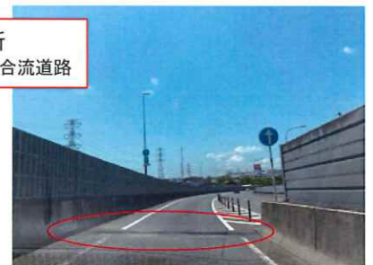
段差補修箇所-2
