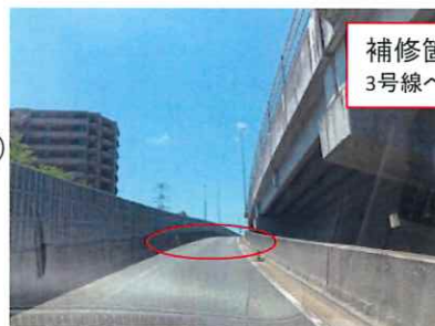
段差補修箇所-1
